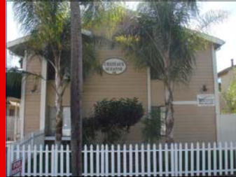
46th Street 14 Units
